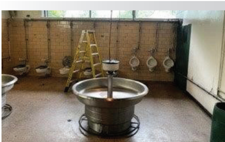
Main Building (Before)
