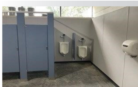
Main Building (Before)
